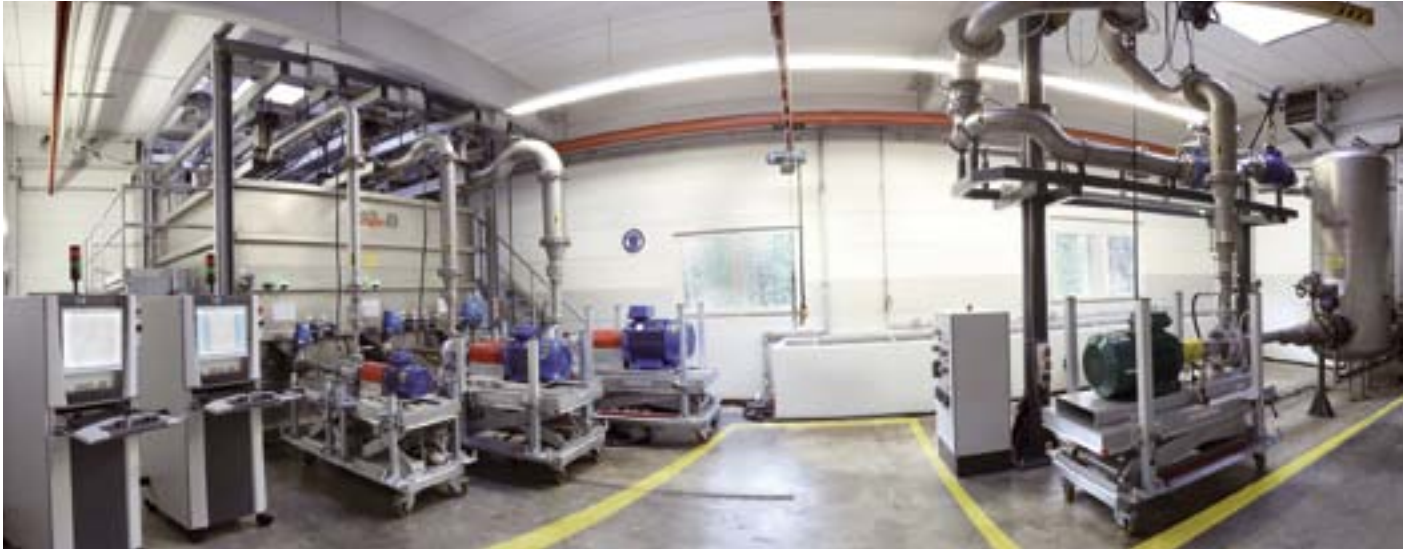
Computer-controlled and fully automated test stands on the premises of Speck in Roth. Measuring of hydraulics, power requirements, axial thrust, vibrations and NPSH values. Heads of up to 400 m and flow rates of up to 750 m 3 /h are possible.
